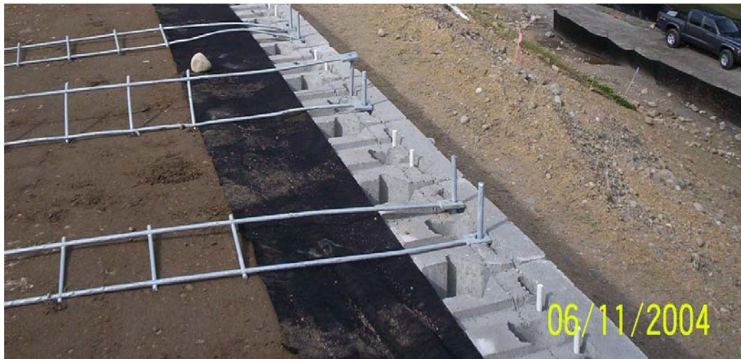
Figure 15-(KeySystem I)-2 KeySystem I wall Keysteel reinforcement connector and block as assembled, showing both fiberglass alignment pins and galvanized steel connector pins.
