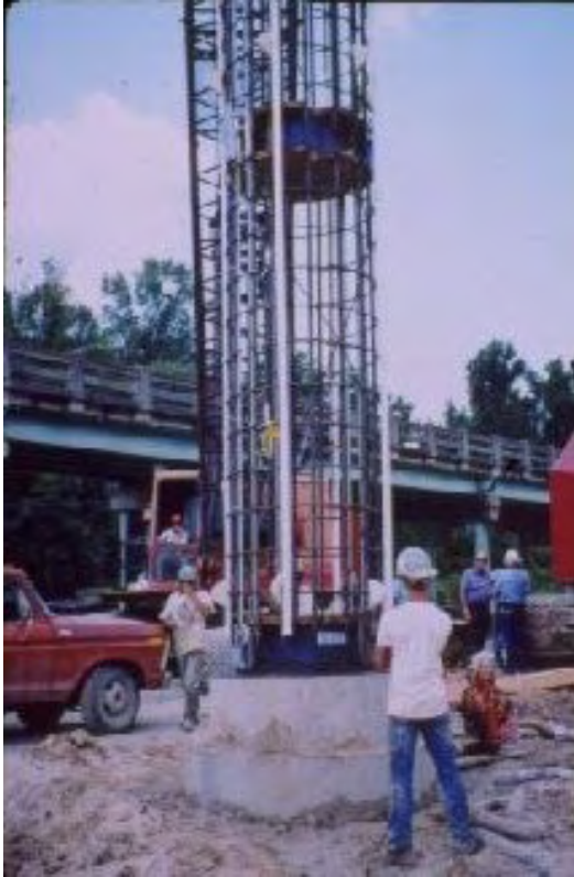
Figure 4142, Osterberg Load Cells
