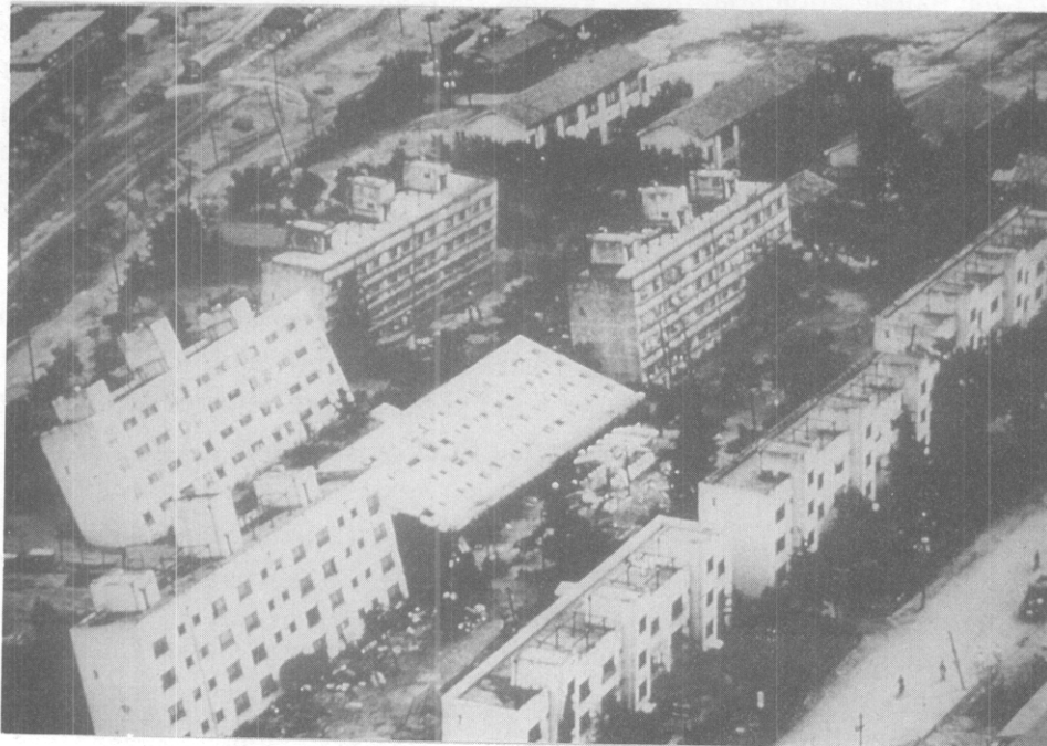
Figure 2. Tilting of buildings due to soil liquefaction during the Niigata (Japan) earthquake of 1964.
