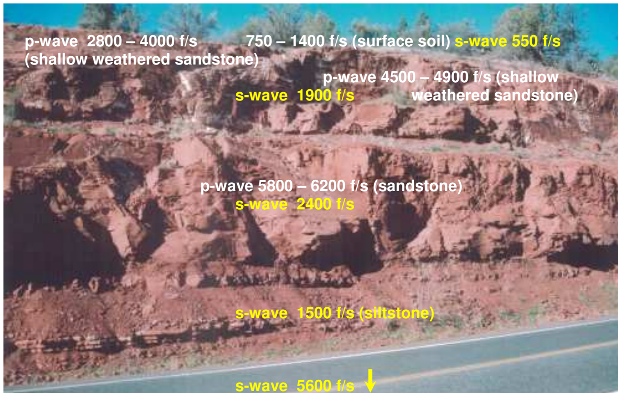
Figure 1. Surface seismic characterization of an existing highway rock cut south of Sedona, Arizona as interpreted from a surface seismic line completed along the top of the cut. This seismic line was one of 60 lines completed as part of the geotechnical investigation for design of major improvements and widening of highway State Route (SR) 179 through a mountainous area near Sedona, Arizona. Interpreted p-wave velocities (in feet per second) at various parts of the exposed rock mass are presented in white. The range of p-wave velocities varies laterally across the cut, but p-wave depth of investigation is limited to the high velocity sandstone horizon. S-wave velocities are presented as a 1-dimensional vertical profile. S-wave characterization includes the less competent slope-forming siltstone material underlying the high velocity sandstone, and a very high velocity horizon underlying the slope toe.
