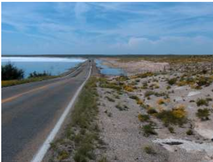
Figure 4. Highway NM 128 crossing into a typical large-scale depression in a regional setting of sedimentary evaporite rock. Evaporite karst is a geologic hazard that impacts the highway in this general area. Seismic data presented in Figures 3, 5, 6 and 7 were collected in the vicinity.
