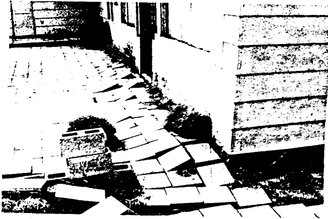
Figure 16. Ground bulging and foundation detachment produced by rotation of the structure's concrete slab.
