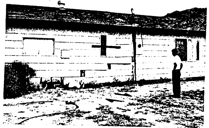
Figure 14. View of the NE side of the house damaged at the Kickapoo Trail site. At the lower left corner, the largest crack (B) is noticeable. Note the influence of the ground rupture extending from the ground, up the wall, and to the roof in the center of the picture.
