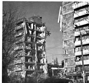
Figure 6.13 Partially collapsed, nine-story residential precast-frame building in Leninakan
