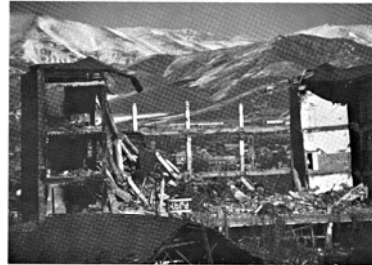
Figure 6.12 Remains of five-story precast-frame communications building in Spitak. It is presumed that the weak floor diaphragms contributed to this failure.
