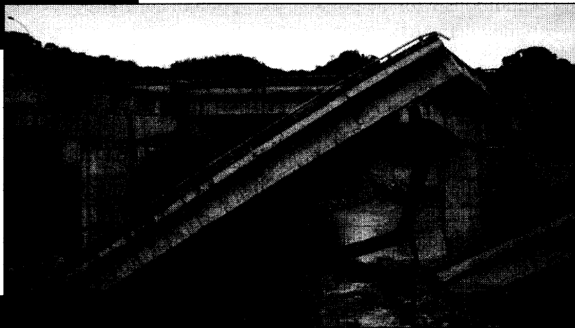
Chi Chi earthquake, 1999
