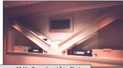
62 Dampers: 30 Kip Capacity, +/-2 in. Stroke
