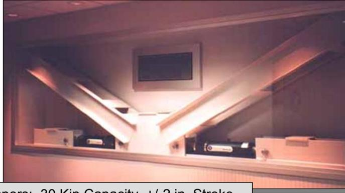
62 Dampers: 30 Kip Capacity, +/-2 in. Stroke
