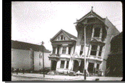
1906 San Francisco Earthquake
