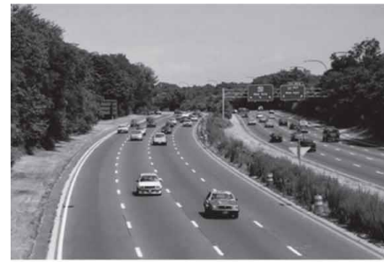
(a) A Typical 8-Lane Freeway
