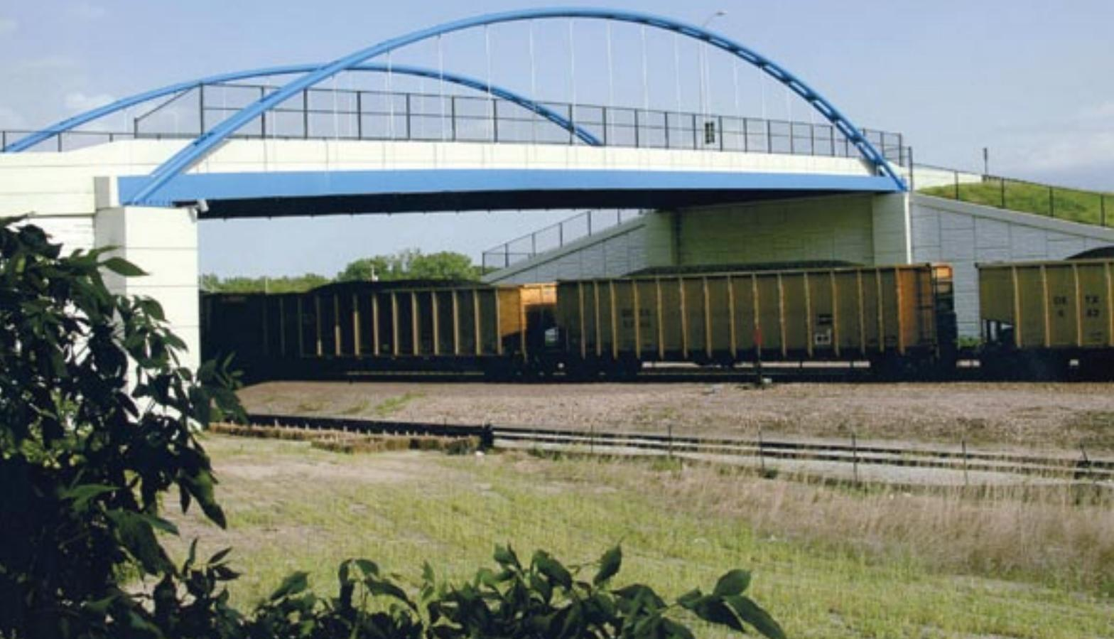
**R**avenna viaduct is located on Highway 68 at the southern edge of downtown Ravenna, Neb. and spans a major route of the Burlington Northern Santa Fe Railroad. The original viaduct, built in 1937, was a five-span 265.5-ft.-long bridge with a 24-ft.-wide roadway and a 5-ft.-wide sidewalk. Thanks to structural deficiency and functional obsolescence, it was replaced with a new 174-ft. single-span parallel tied arch viaduct with a 43-ft.-wide roadway and 8-ft.-wide sidewalk.
