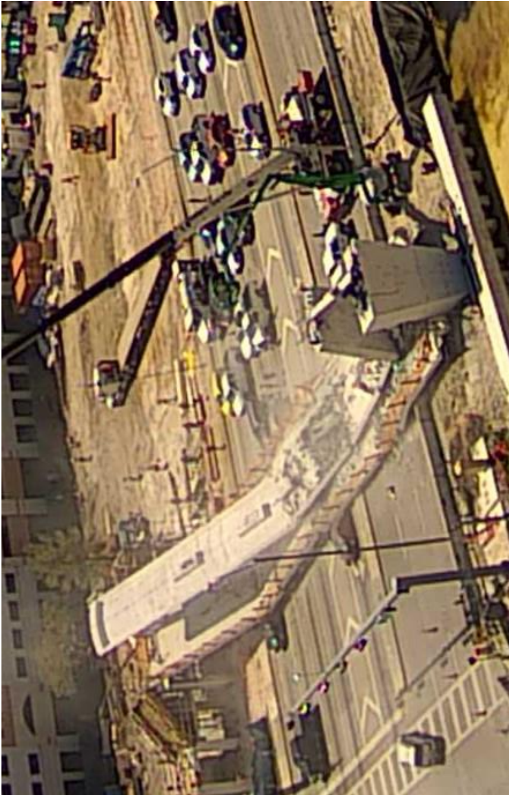
Figure 49 Bridge immediately after the collapse, March 15, 2018 – camera #2 Employees engaged in re-tensioning the PT bars in diagonal 11
