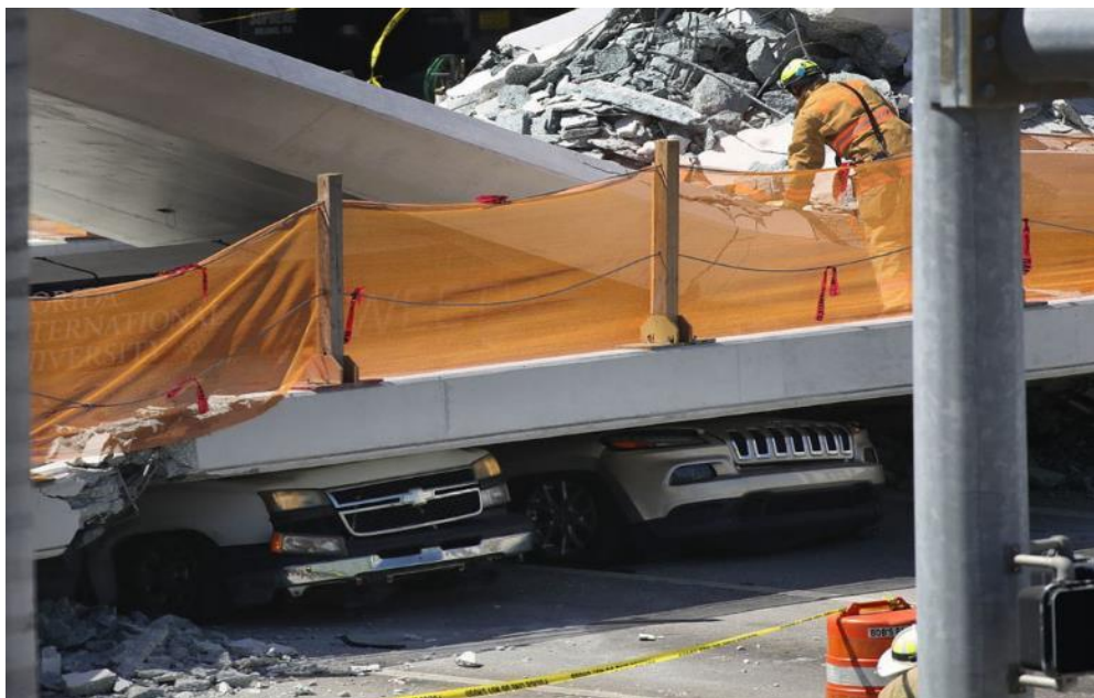
Figure 75 Vehicles crushed by falling bridge
