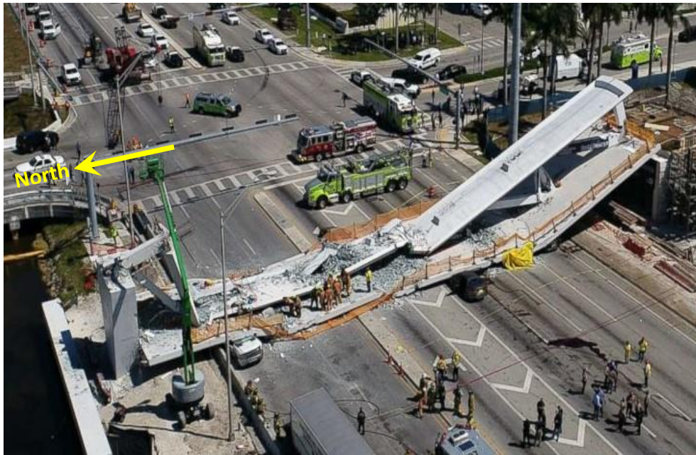
Figure 72 Aerial view of the collapsed bridge, March 15~18, 2018
