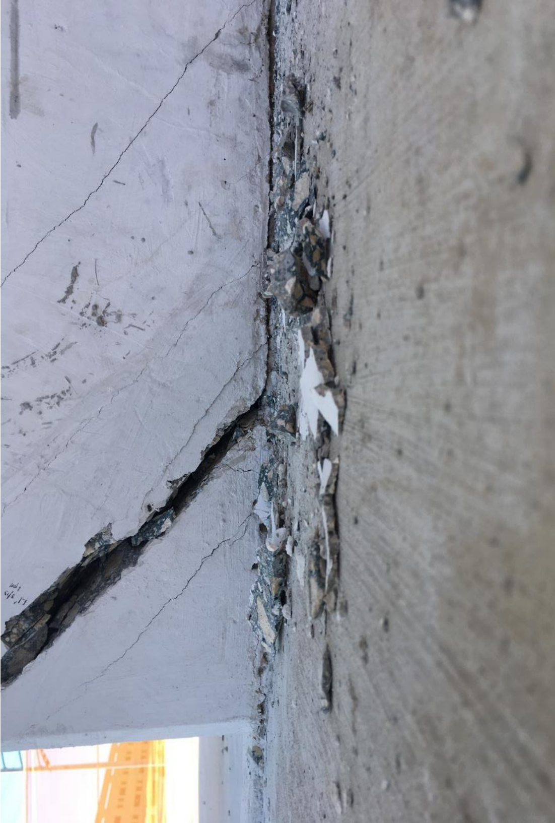
Figure 35 Cracks at the construction joint of the main span deck, diagonal 11 and the chamfer of diagonal 11 on 3/13/2018 by BPA
