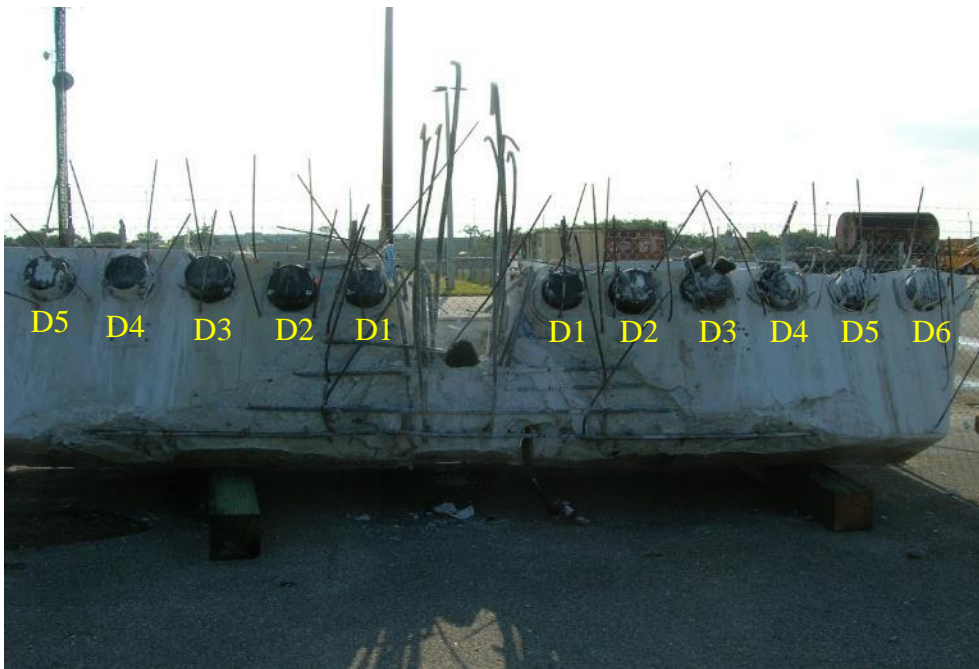
Figure 61 Remnants of diaphragm II at the time of the bridge collapse in the storage yard – looking north from south, April 9, 2018, by OSHA
