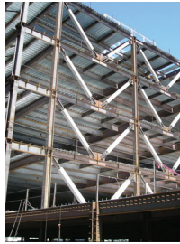
diagonal bracing
