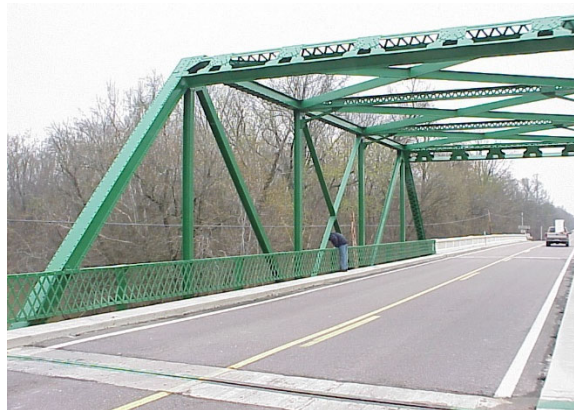
Figure 2. Truss bridge in West Tennessee.
