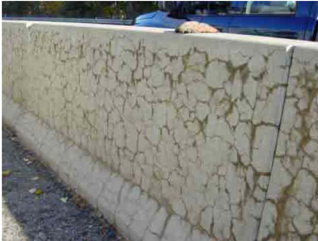
Map Cracking
