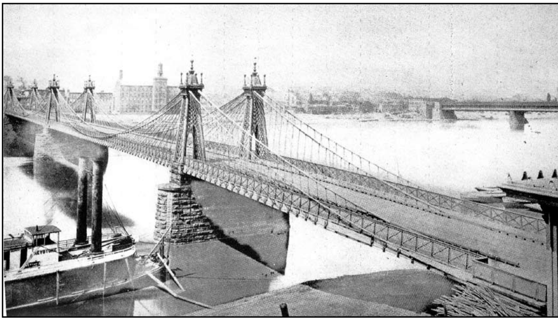
Allegheny River Bridge 1860 to 1891
