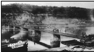
Smithfield Street Bridge Monongahela River Pittsburgh 1846
