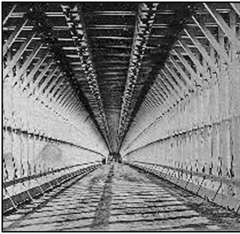
Niagara lower deck and side trusses
