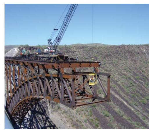
provide support and anchorage for the cantilever launch of the steel arch over the canyon. Flexible connection details were provided for ease of fabrication, transport, and field erection.
