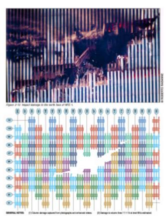
Figure 5: Damage to North Face of WTC 1 (Source: FEMA report)
