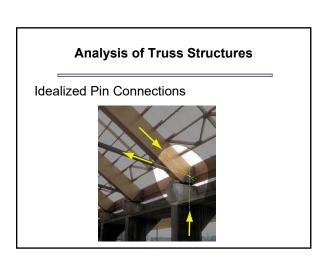
➤ Typically, the joint connections are formed by bolting or welding the end members together to a
