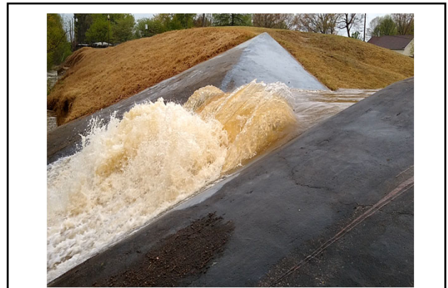
On Sunday, April 7, 2019, another significant rainfall required the Yale Road detention pond to be utilized (video).
