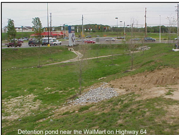
Detention pond near the WalMart on Highway 64
