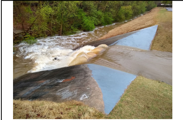
On Sunday, April 7, 2019, another significant rainfall required the Yale Road detention pond to be utilized.
