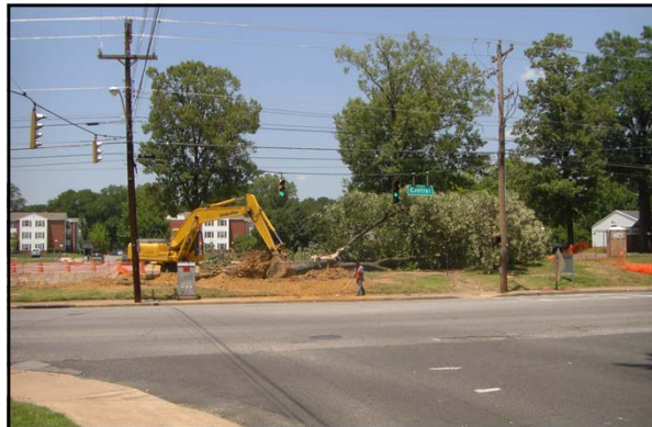
In the summer 2011, a new underground detention pond was constructed under the Central parking at the University of Memphis
