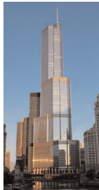
Figure 19-8. Completed in 2009, the 92 story Trump International Hotel and Tower, which was constructed with high-performance SCC, is the tallest building (at 1170 ft [1389 ft to the top of the spire]) built in North America since the completion of the Sears Tower in 1974.
