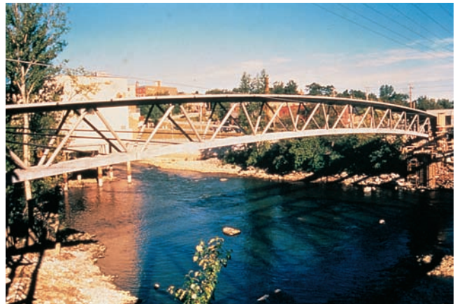
Figure 19-10. The Sherbrooke footbridge in Quebec, built in 1997, is North America's first reactive-powder ultra-high performance concrete structure.
