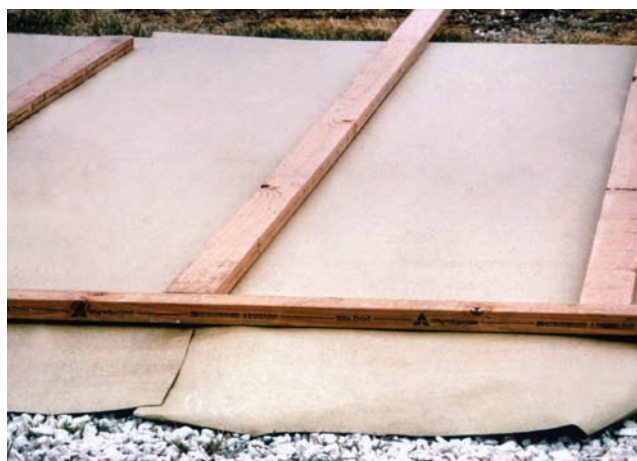
Figure 15-6. Impervious curing paper is an efficient means of curing horizontal surfaces.
