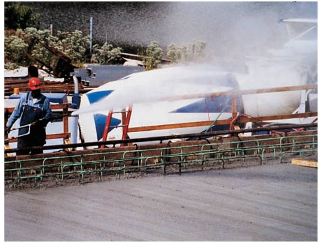
Figure 15-4. Fogging minimizes moisture loss during and after placing and finishing of concrete.
