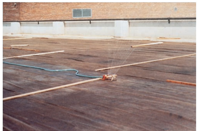
Figure 15-5. Lawn sprinklers saturating burlap with water keep the concrete continuously moist. Intermittent sprinkling is acceptable if no drying of the concrete surface occurs.
