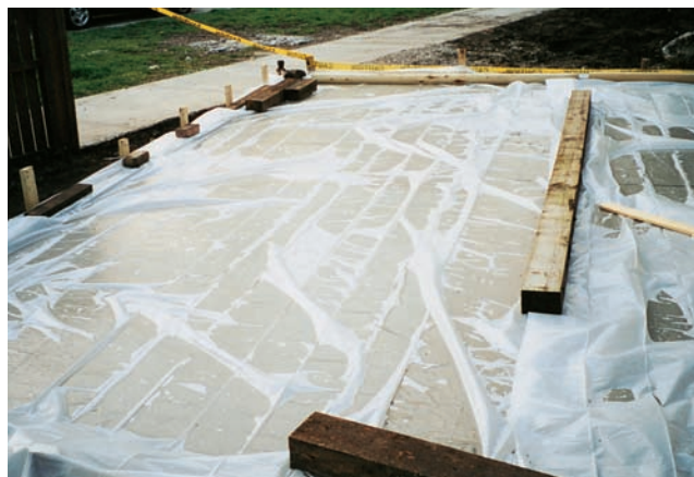
Figure 15-7. Polyethylene film is an effective moisture barrier for curing concrete and easily applied to complex as well as simple shapes. To minimize discoloration, the film should be kept as flat as possible on the concrete surface.
