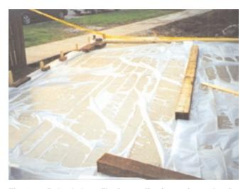
Fig. 12-7. Polyethylene film is an effective moisture barrier for curing concrete and easily applied to complex as well as simple shapes. To minimize discoloration, the film should be kept as flat as possible on the concrete surface. (70014)
