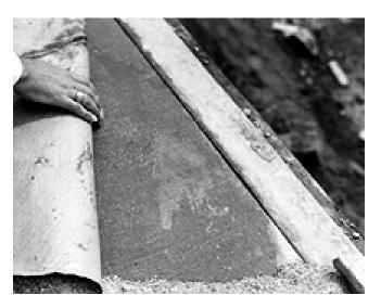
Fig.12-6. Impervious curing paper is an efficient means of curing horizontal surfaces. (69994)
