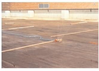
Fig. 12-5. Lawn sprinklers saturating burlap with water keep the concrete continuously moist. Intermittent sprinkling is acceptable if no drying of the concrete surface occurs. (50177)
